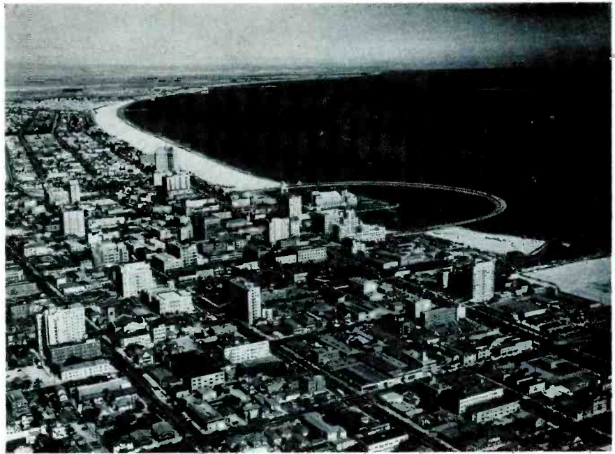
Aerial view showing Long Beach Harbor with Municipal Auditorium inside horseshoe —Pacific Air Industries Photo.
